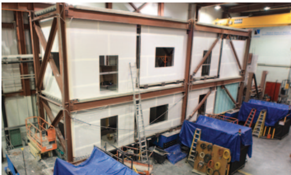
Fig. 1.2 NEESR-GC: simulation of the seismic performance of nonstructural systems. NSF Award #: 0721399PI: Emmanuel “Manos” Maragakis. Co-PIs: Robert Reitherman, Steven French, Andre Filiatrault, Tara Hutchinson. Research Sites: University of Nevada, Reno; Hyogo Earthquake Engineering Research Center, aka “E-Defense,” Miki, Japan; NEES, University at Buffalo. (Reproduced by permission of PI: Emmanuel “Manos” Maragakis, Dean of Engineering, University of Nevada, Reno)
