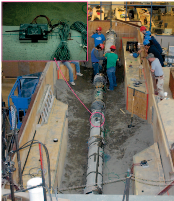
Fig. 1.4 NEESR-SG: damage detection and health monitoring of buried pipelines after earthquake-induced ground movement. NSF Award #: 0724022. PI name: Radoslaw Michalowski. Co-PIs: W. Jason Weiss, Russell Green, Jerome Lynch, Aaron Bradshaw Research Site: Cornell. (Reproduced by permission of PI: Radoslaw Michalowski, Department of Civil and Environmental Engineering, University of Michigan)
