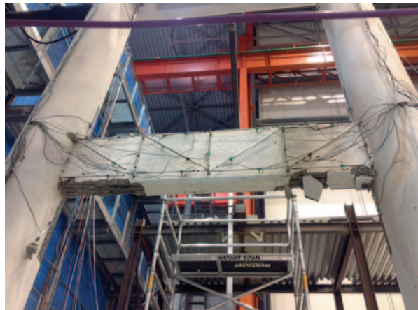
Fig. 14.16 Transverse beam damage on pier 11 after test k12 (PGA=200% ULS)
