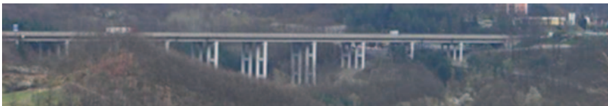
Fig. 13.1 General view of the viaduct Rio-Torto
