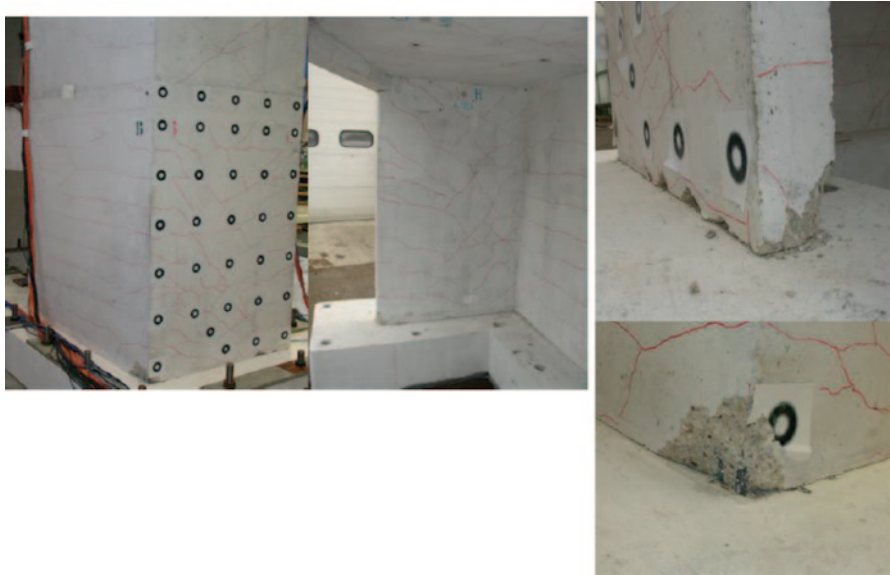
Fig. 19.16 Damage observed on wall 1 after 0.8 g tests
