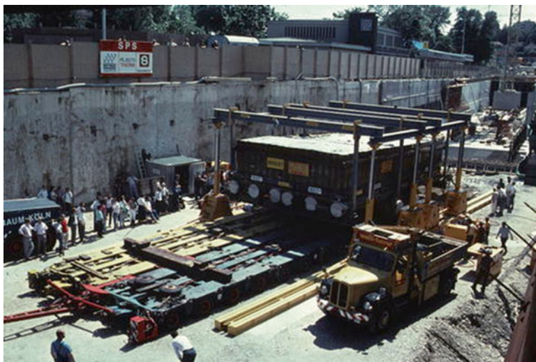
Fig. 20.4 Transport of a portion of a Magdalenian open-air site. This unusual operation was entirely financed by the Swiss Federal Roads Office (© photo Y. André, Office et Musée d'archéologie Neuchâtel)
