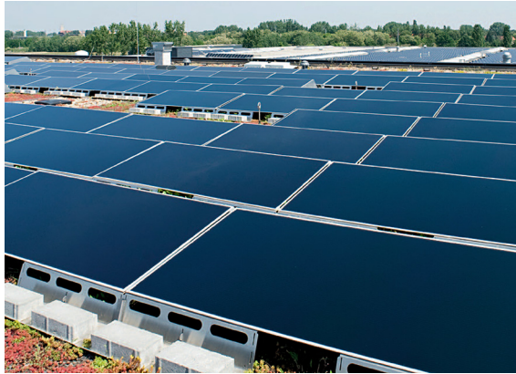
Fig. 6 Tectum flat roof system
