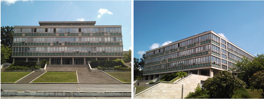
Fig. 7 Picture of the dormitory building
