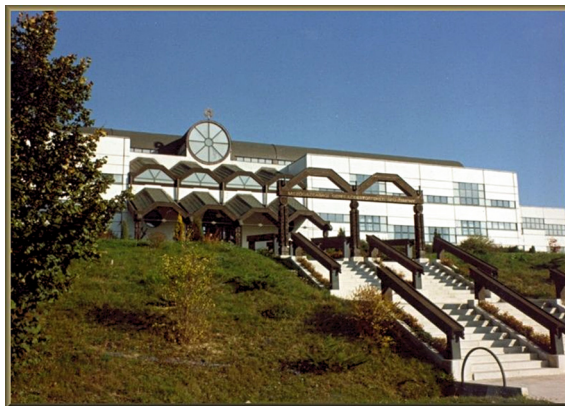
Fig. 5 Picture of the knowledge transfer centre building
