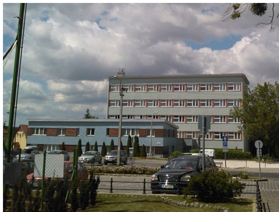
Fig. 4 Picture of the dormitory building
