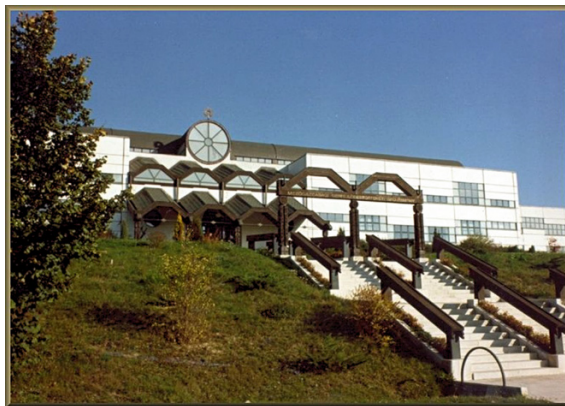
Fig. 5 Picture of the knowledge transfer centre building
