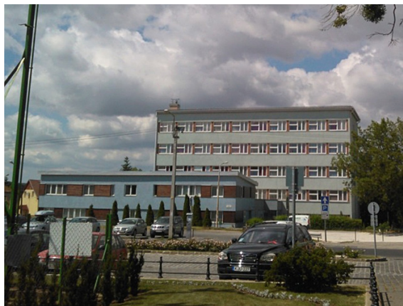
Fig. 4 Picture of the dormitory building
