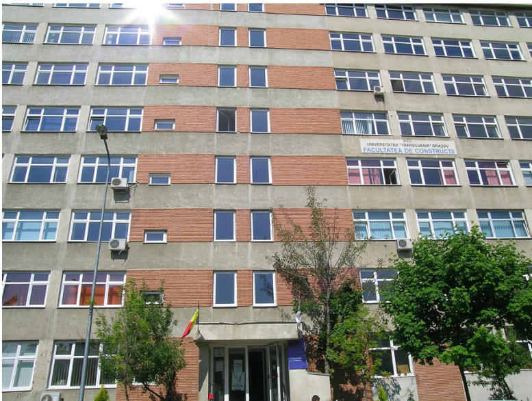
Fig. 1 Overview of the studied building
