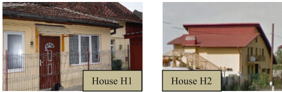
Fig. 2 The two residential buildings H1 (Brasov) (left) and H2 (Bucharest) (right) [6]
