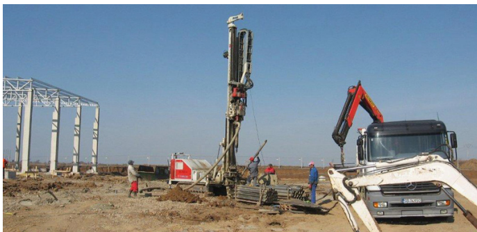
Fig. 1 The drilling process for the vertical earth loops
