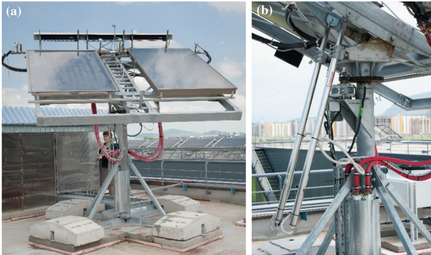
Fig. 11 Tracked platform with solar—thermal flat plate collectors: a general view and b biaxial, azimuthal tracking mechanism
