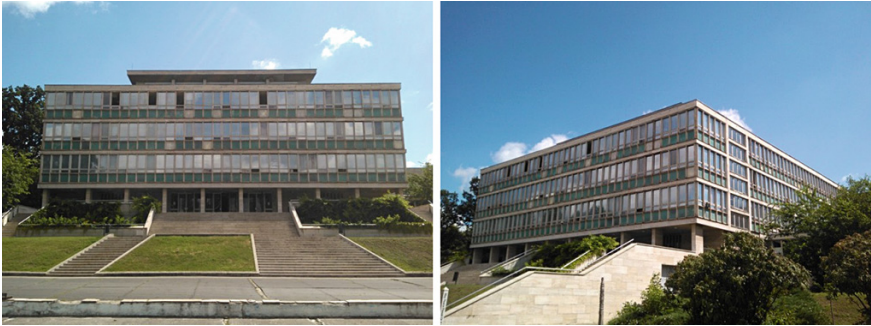
Fig. 7 Picture of the dormitory building
