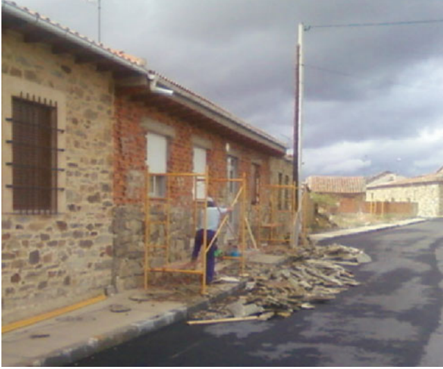
Fig. 3.1 A man gets rid of the stones covering his brick and concrete modern house
