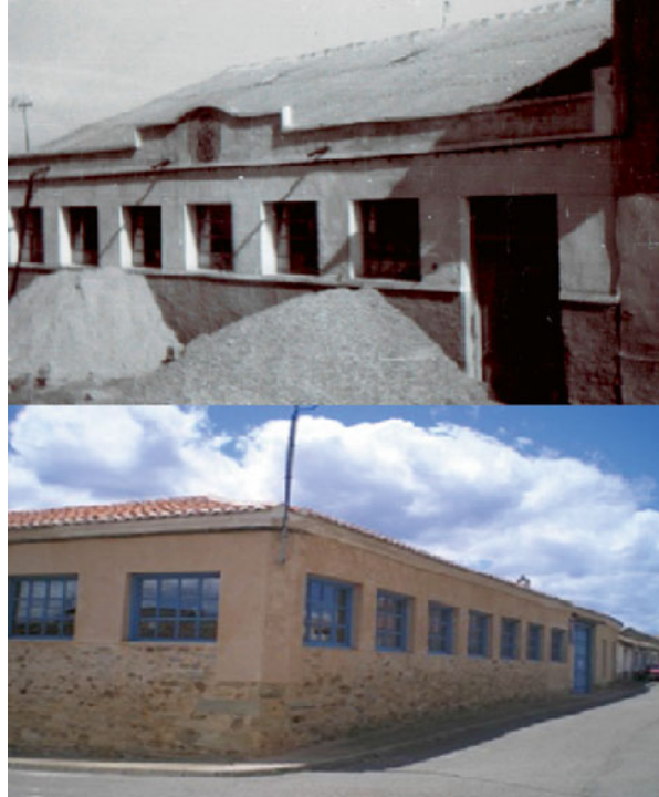
Fig. 3.5 The aspect of La Comunal as a factory with fiber cement roof and concrete in sight ( above ) and as a heritagized entity made of artisan tiles and painted with “traditional” colors. Now, stones are on sight while concrete has been covered ( below )
