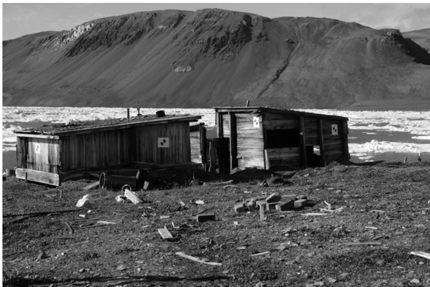
Fig. 11.2 Robert Peary's hut complex reflecting basic principle of Inughuit (Polar Eskimo) architecture
