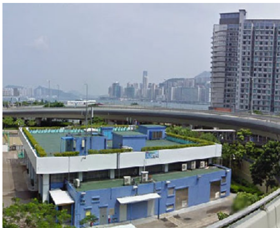
Fig. 8 Pilot sites for PAS55 implementation—Hung Hom Bay sewage pumping station
