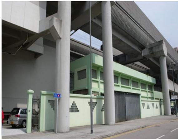
Fig. 7 Pilot sites for PAS55 implementation—Ho Pong street sewage pumping station
