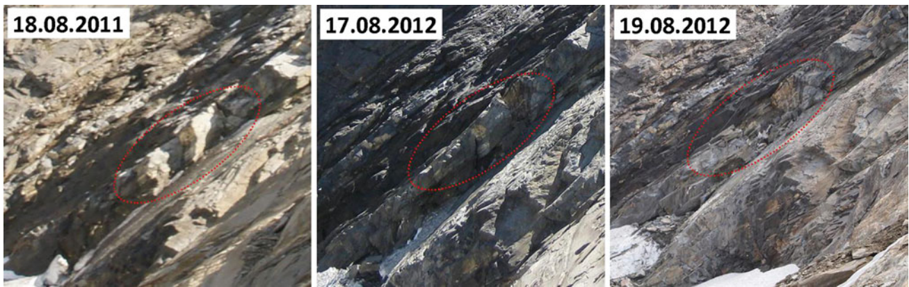
Fig. 48.3 Detachment of the blockslide: 18 August 2011 ( left )—intact rock, 17 August 2012—crack visible in the tensile zone ( middle ), 19 August 2012—situation after the release ( right )
