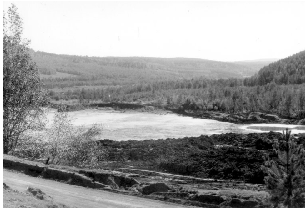
Fig. 54.2 Sludge storage (Darasun gold deposit, Eastern Transbaikalia)
