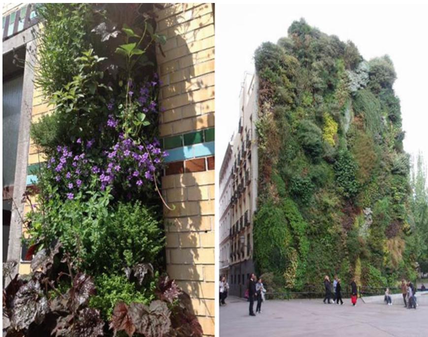
Fig. 6.17 Left photo example of a living wall (felt layers) attached to a façade in the inner city of Antwerp (Belgium). Right photo living wall system in the inner city of Madrid (Spain)
