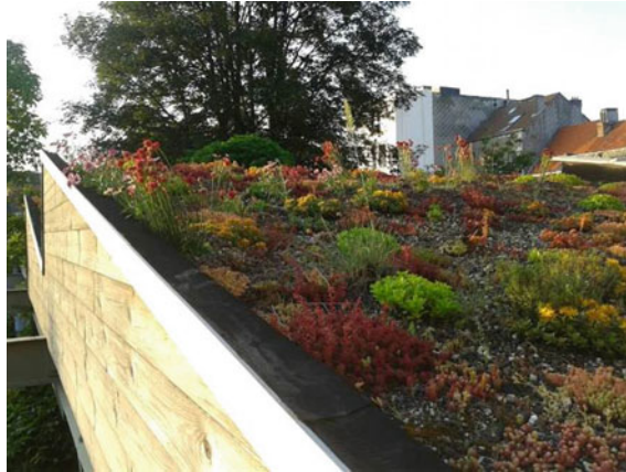
Fig. 6.8 Extensive sloped green roof (Berghem, Belgium)
