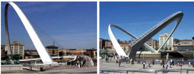
Fig. 10.9 Gateshead Millennium bridge (Hu et al. 2013)
