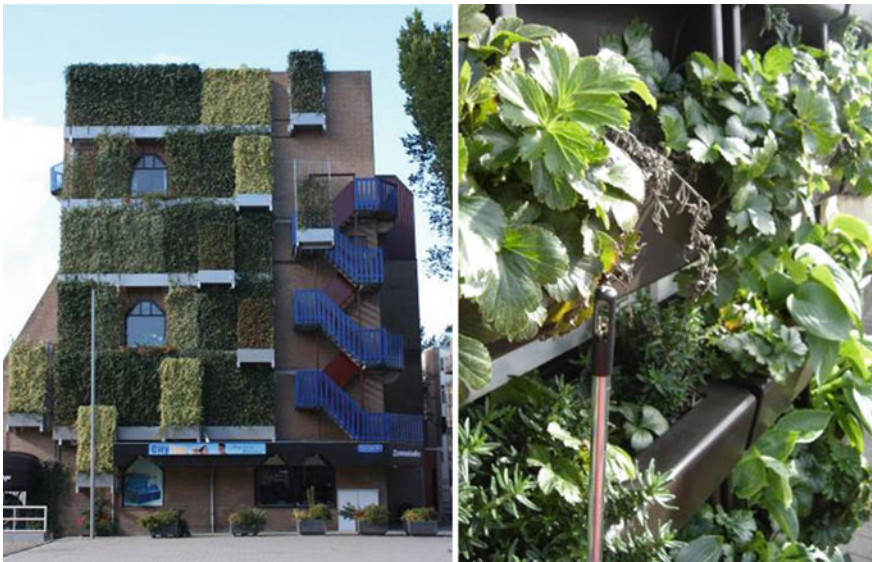
Fig. 6.14 Left indirect greening system based on climbing plants attached to the façade in planter boxes. Right planterboxes system filled with small shrubs
