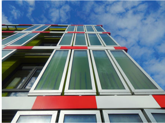
Fig. 5.4 Algae facade, BIQ house at the International Building Exhibition 2013 in Hamburg (Source http://www.flickr.com/photos/_bundjugend/ under CC BY 2.0 license)
