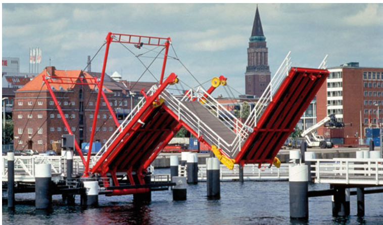
Fig. 10.10 Folding bridge at Kiel ( photo Schlaich Bergemann and Partner)
