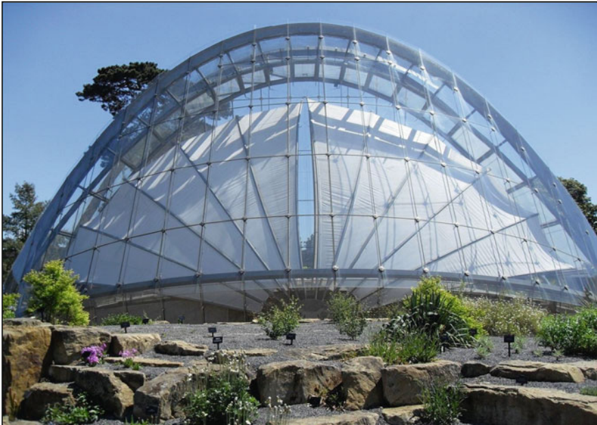
Fig. 4.3 Davis alpine house, London, England (photo by P. Galletly)
