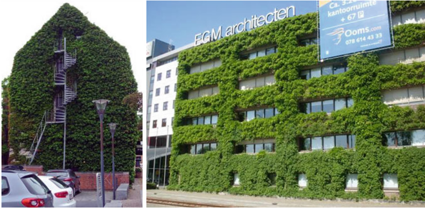
Fig. 6.13 Examples of green facades (rooted into the ground) left photo Dordrecht (The Netherlands), right photo Frederikshaven (Denmark)
