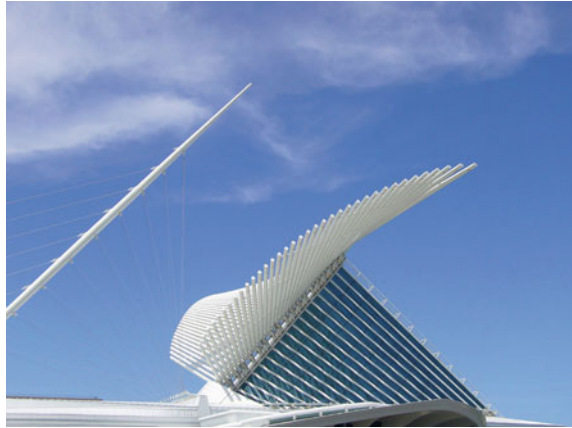
Fig. 5.3 Burke Brise Soleil at the Milwaukee Art Museum. Architect: Calatrava (Source http://www.flickr.com/photos/crazyegg95/ under CC BY-ND 2.0 license)
