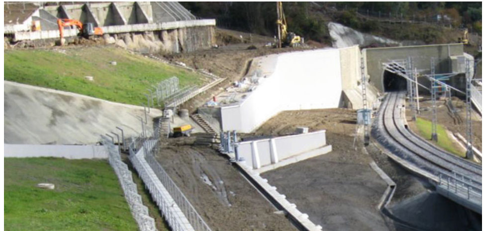
Fig. 370.2 General view on the constructed railway tunnel and pre-portal construction
