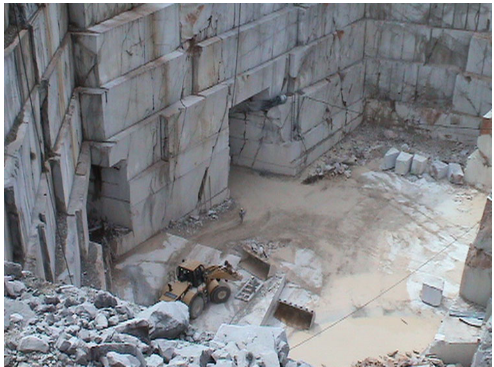
Fig. 43.3 South portal face wall with the entrance into Lipica II quarry underground galleries (Kortnik 2012)
