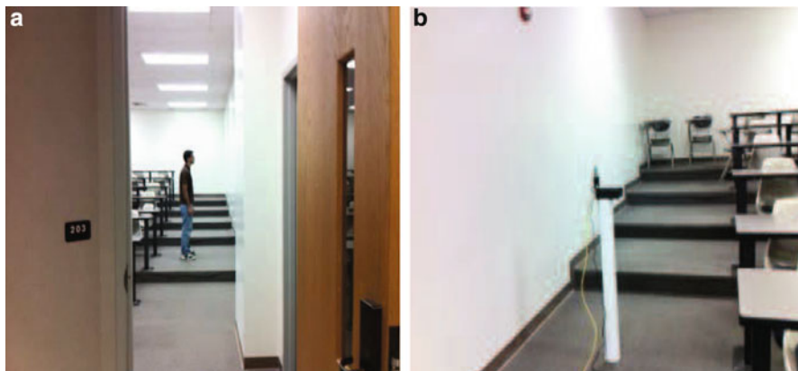
Fig. 16.2 Location of the human target and UWB radar on different sides of a 1 ft thick Gypsum partition wall (a) human target and (b) UWB radar
