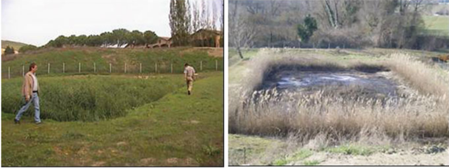
Fig. 13.2 The initial 500 m 2 HF CW before ( left ) and after ( right ) the occurrence of severe clogging generated by progressively increasing overloading of the system
