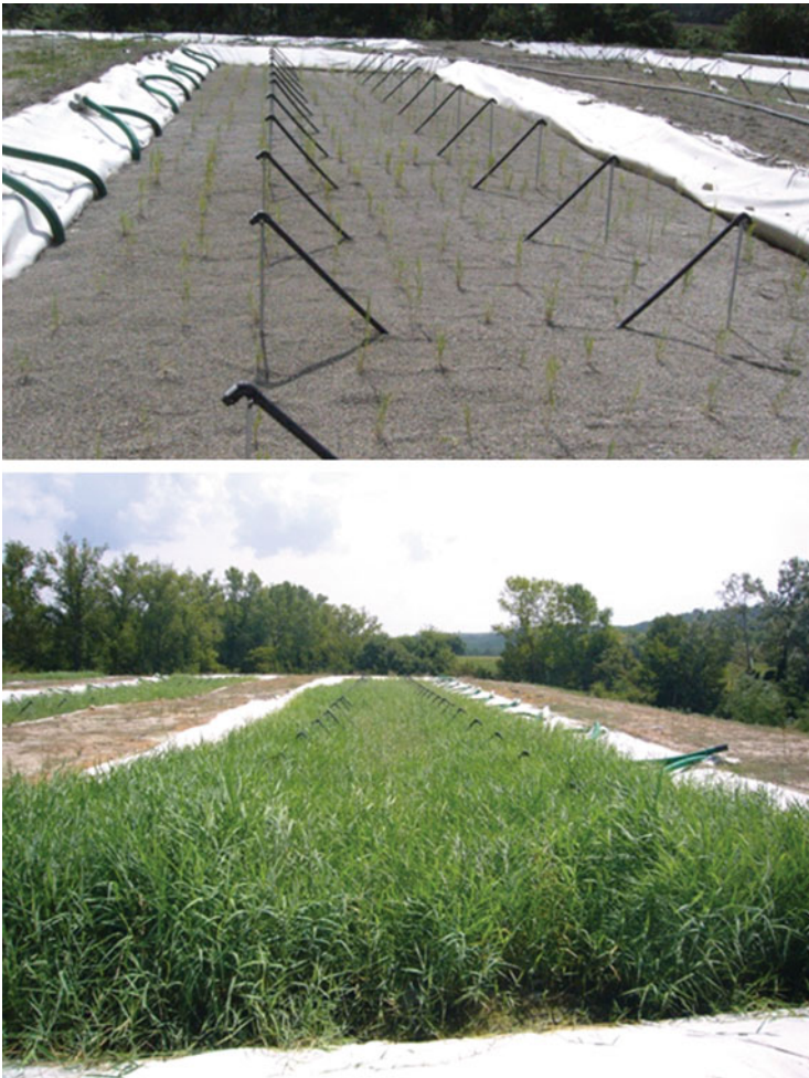
Fig. 13.3 RBF at the plantation time ( top ) and after 1 year of operation ( bottom )
