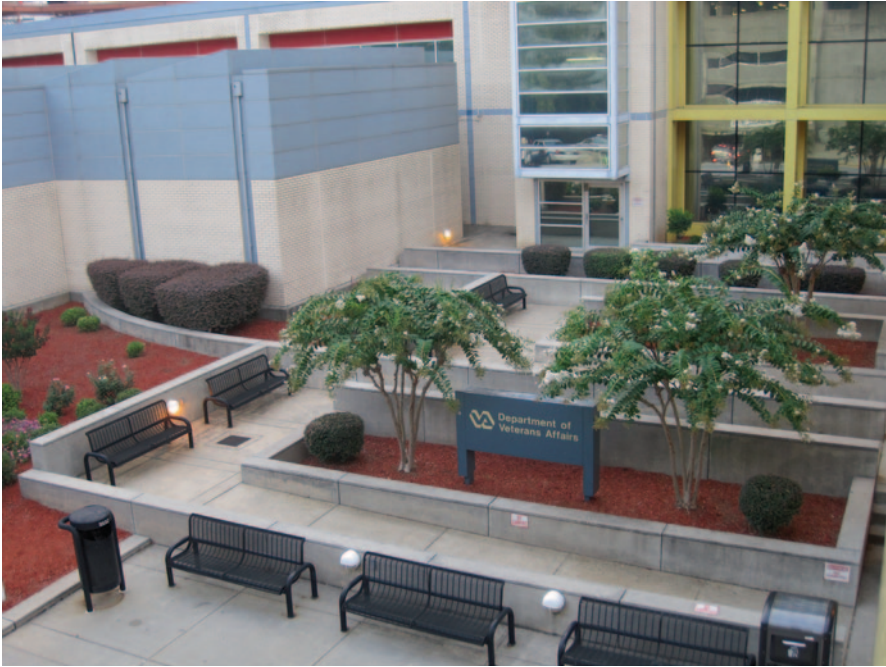
Fig. 24.1 Sloping walkways that are integrated into landscape and have well-defined edges (e.g., low walls and planters). These enable all users to get to the entrance in the same manner. These features exemplify principles: P1. Equitable use, P2. Flexibility in use, P4. Perceptible information; P6. Low physical effort, P7. Size and space for approach and use, P8. Social integration and P9. Contextual integration
