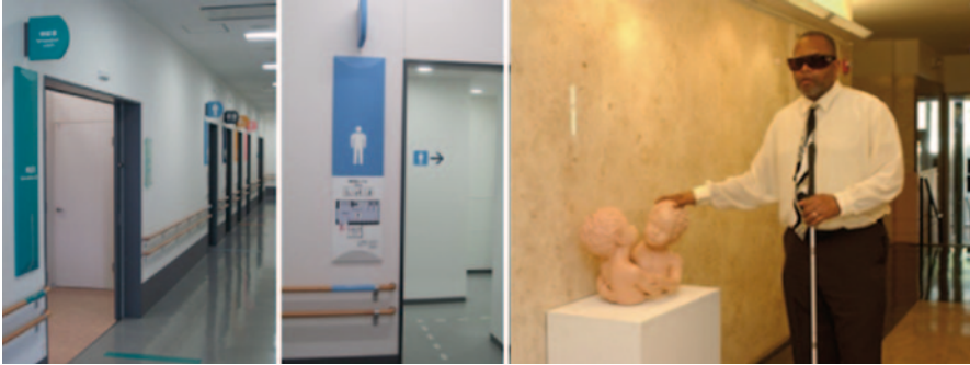
Fig. 24.4 Redundant and multisensory way-finding systems, including color changes in signs and floor colorings as well as tactile information on wall and handrail signs exemplify principles: P1. Equitable use, P2. Flexibility in use, P3. Simple and intuitive use, P4. Perceptible information; P5. Tolerance for error, P8. Social integration, and P9. Contextual integration
