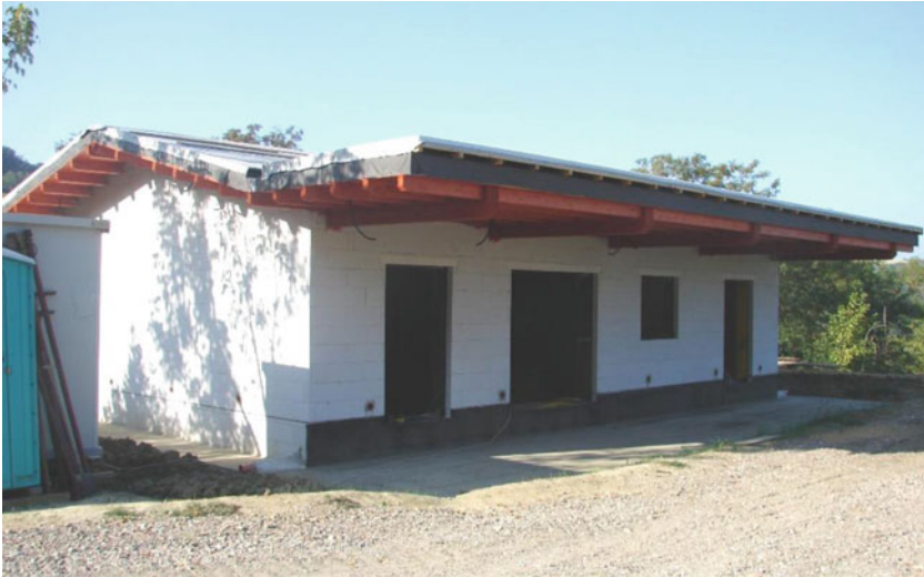
Fig. 12.2 View of the North side of the house (under construction)
