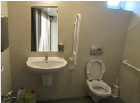
Fig. 10 The accessible toilet finished
