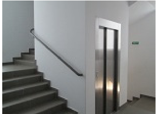
Fig. 7 The finished elevator cage
