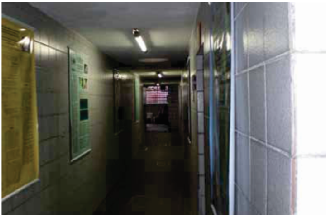
Fig. 3. The lighting is precarious in the corridors
