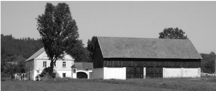
Fig. 3. Multi-house enclosed homesteads with an internal farmyard and a shrine at the entrance (Oldrychowice), (photo by E. Trocka-Leszczynska, 2009)
