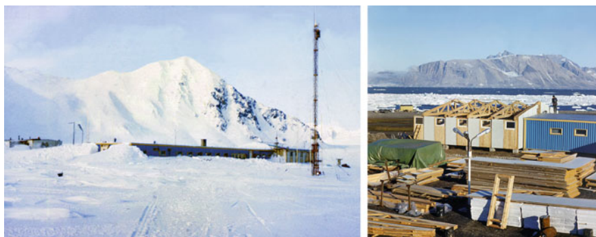
Fig. 3 Left view on the Polish Polar Station Hornsund in Isbjørnhamna Bay in the 1980s. Right construction works on the so-called summer base in the summer of 1979
