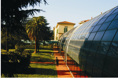
Fig. 4. Courtyard and the main entrance to Children's Hospital in Florence (photo. Magdalena Jamrozik-Szatanek)
