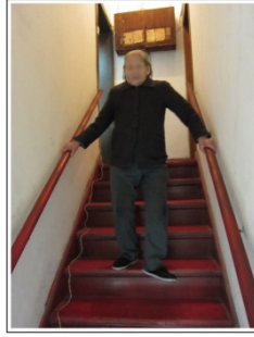
Fig. 5. The stair with wood armrest
