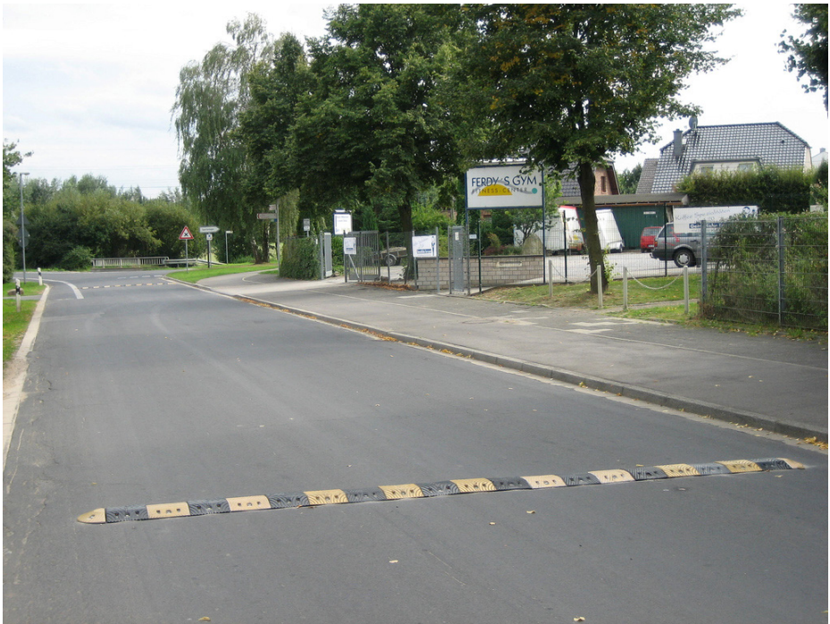
Fig. 6. Speed bump forcing drives to slow down or feel discomfort (Photo by Marco: http://flic.kr/p/5iqxpN )
