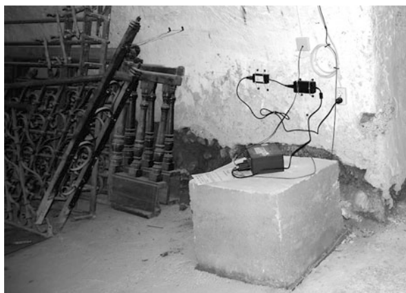
Fig. 5.3 The accelerometric station in the basement of the old jailhouse, Lorca
