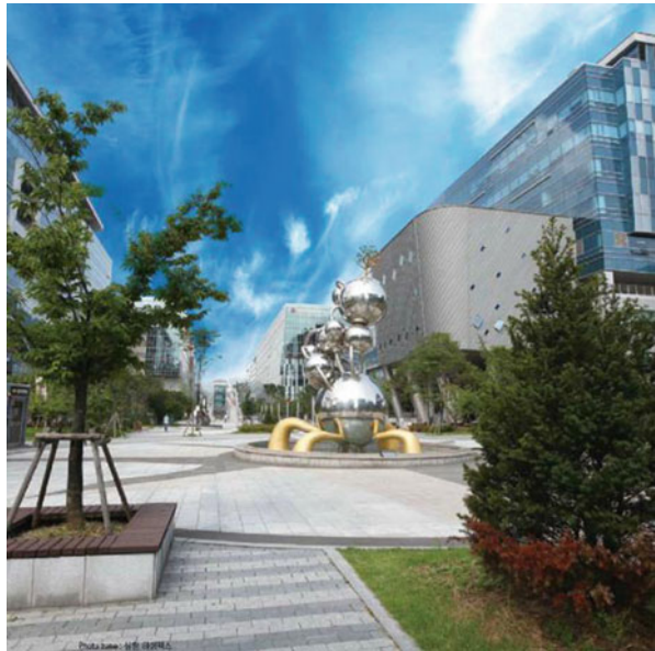
Fig. 2 New buildings in Pangyo Techno Valley
