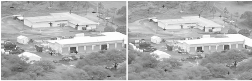
Fig. 5 The aerial image set, representing two aerial images captured from different views and distances of a few buildings
