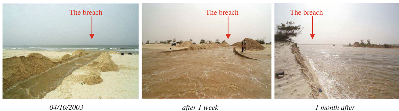
Photo 2 Progression of the gap between October and November 2003 (Photos 1. Diop, 2003)
