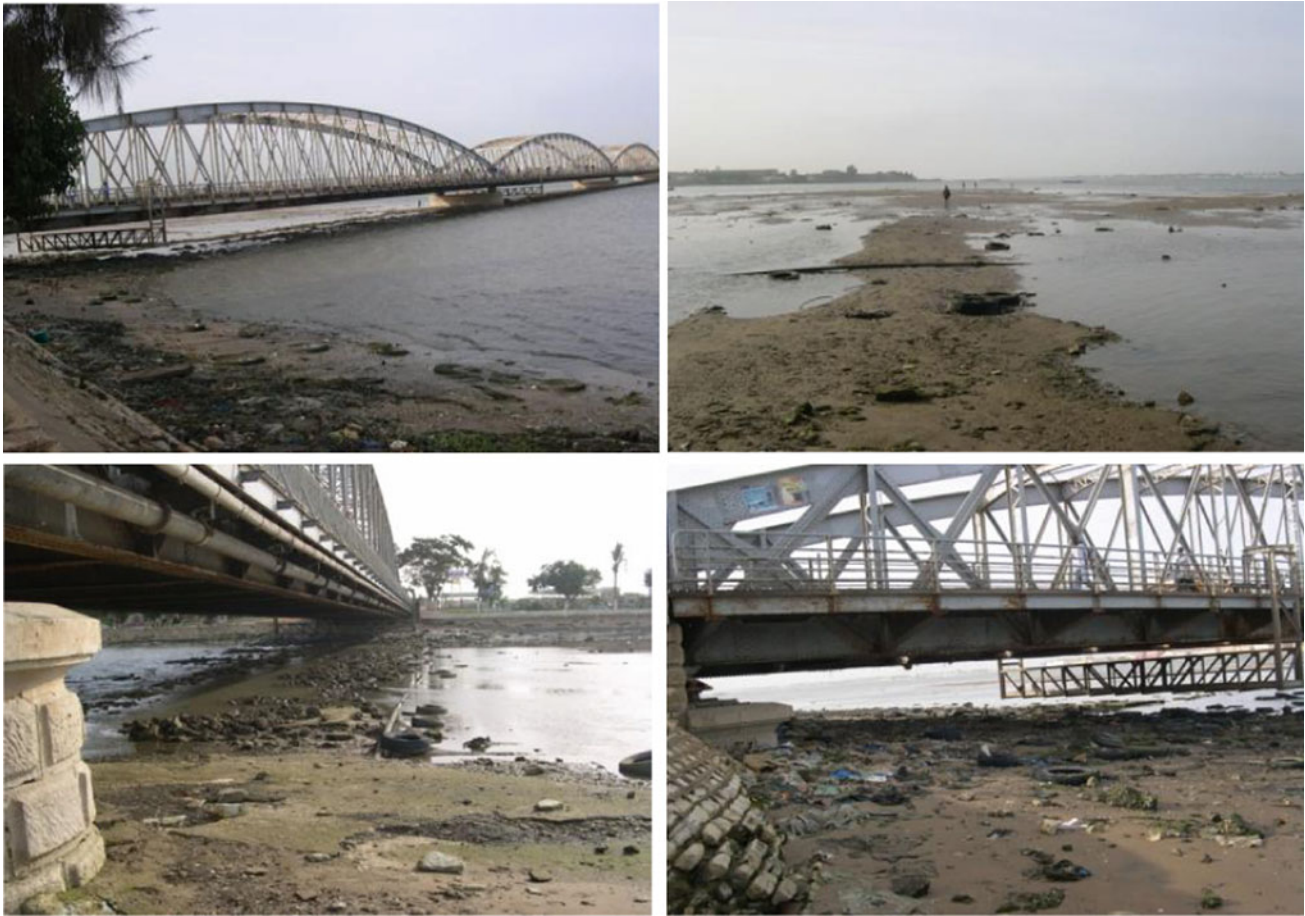
Photo 3 Withdrawal of the Senegal river at low tide at the Faidherbe bridge (Pictures from Kane A., December 2003)
