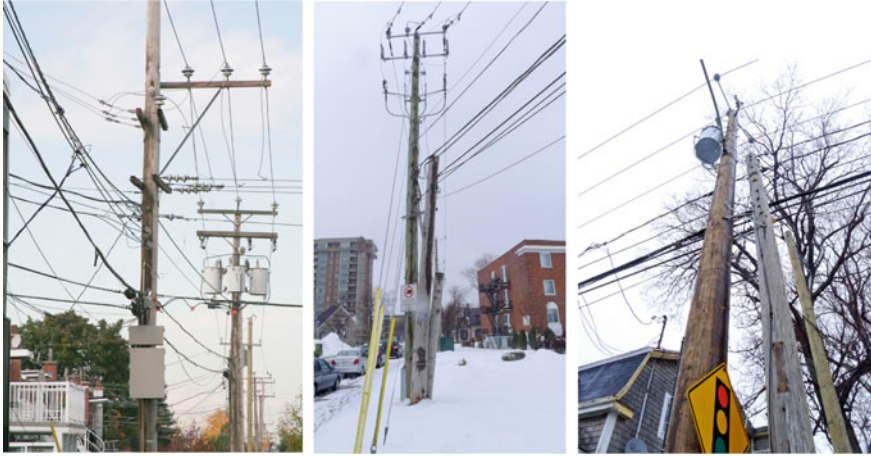
Fig. 1 Examples of saturation and the coexistence of old and new structures
