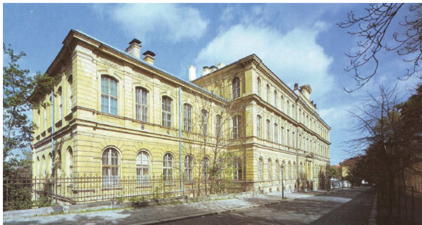
Fig. 1 The building of the former Faculty of Philosophy of the German University on Viničná 7 wherein Einstein had “an excellent Institute with a beautiful library”
