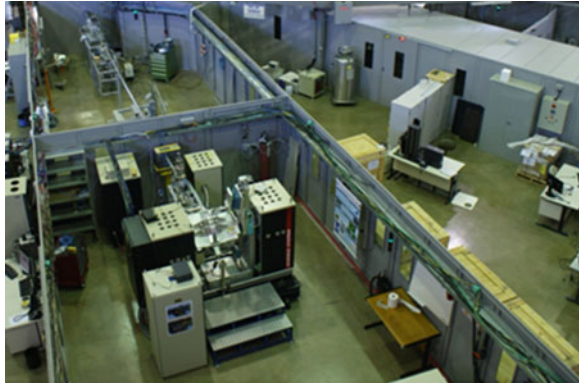
Fig. 1 XTMS installation at the Brazilian Synchrotron Light Laboratory (LNLS) experiment hall
