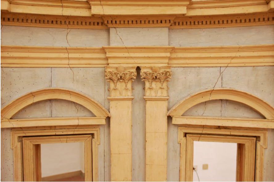
Fig. 3 Detail of the wooden model of Michelangelo's dome, showing painted "cracks" in the structure by Luigi Vanvitelli
