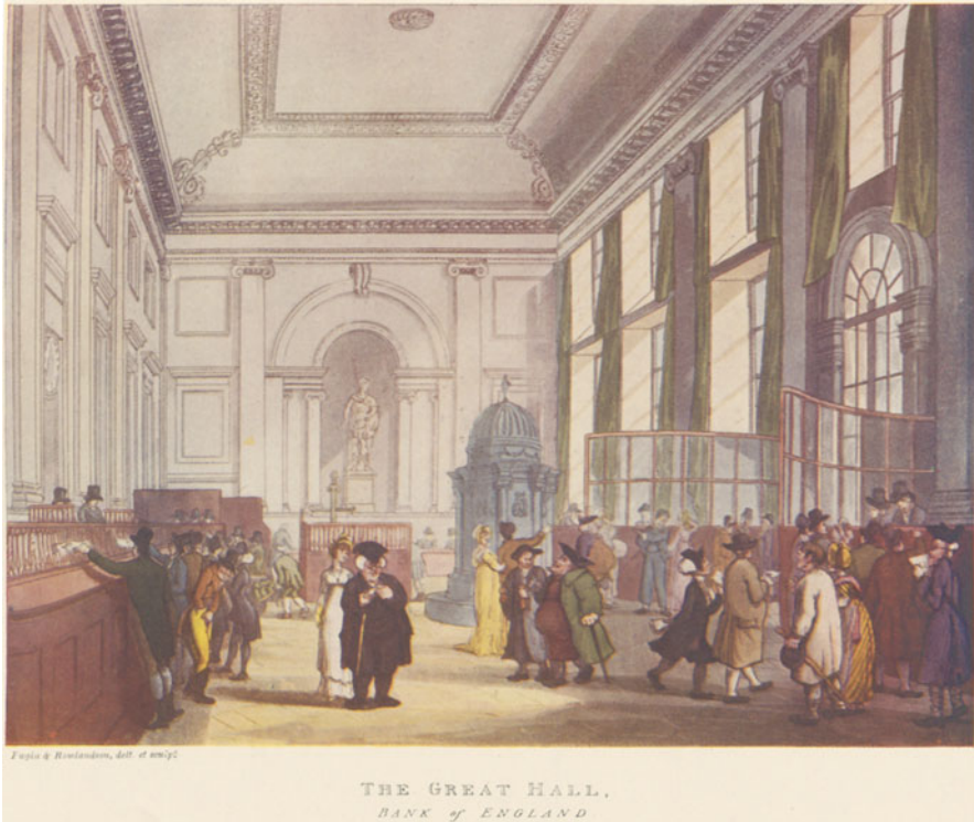
Fig. 14 Interior view of John Soane's Bank of England. The blue domed structure is the closed stove which is supplied and exhausted by underfloor flues (From [Pyne and Combe] 1904)
