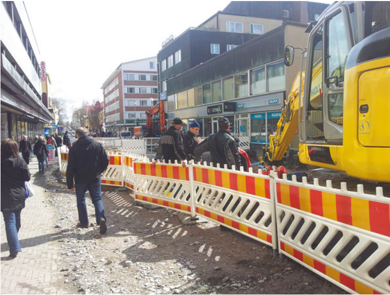
Fig. 7.1 One of the walking streets being renovated
