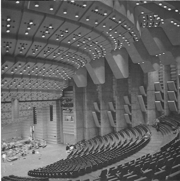
Fig. 2.4 Grieghallen in Bergen, one of the first concert halls where computerized ray tracing was used as a design tool
