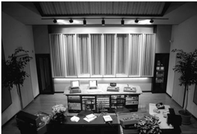
Fig. 6.8 Gateway Mastering, Portland, ME showing a fractal diffusing rear wall (Diffractal ® ). (Photo courtesy of Gateway Mastering + DVD)
