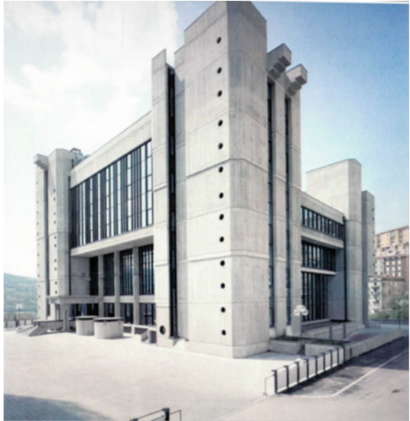
Fig. 11.1 View of the North-East tower
