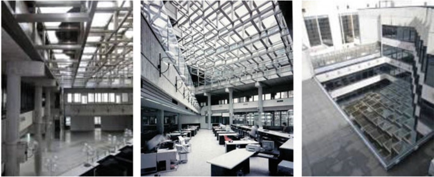
Fig. 11.3 Views of the central atrium glass roof
