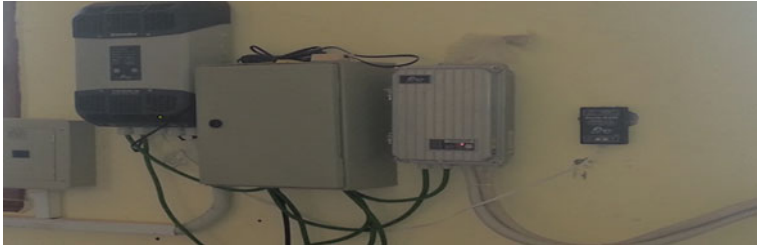
Fig. 46.3 From right to left (Xcom-232i data logger, Vario Track charge controller, combination box, Xtender inverter, switches box)
