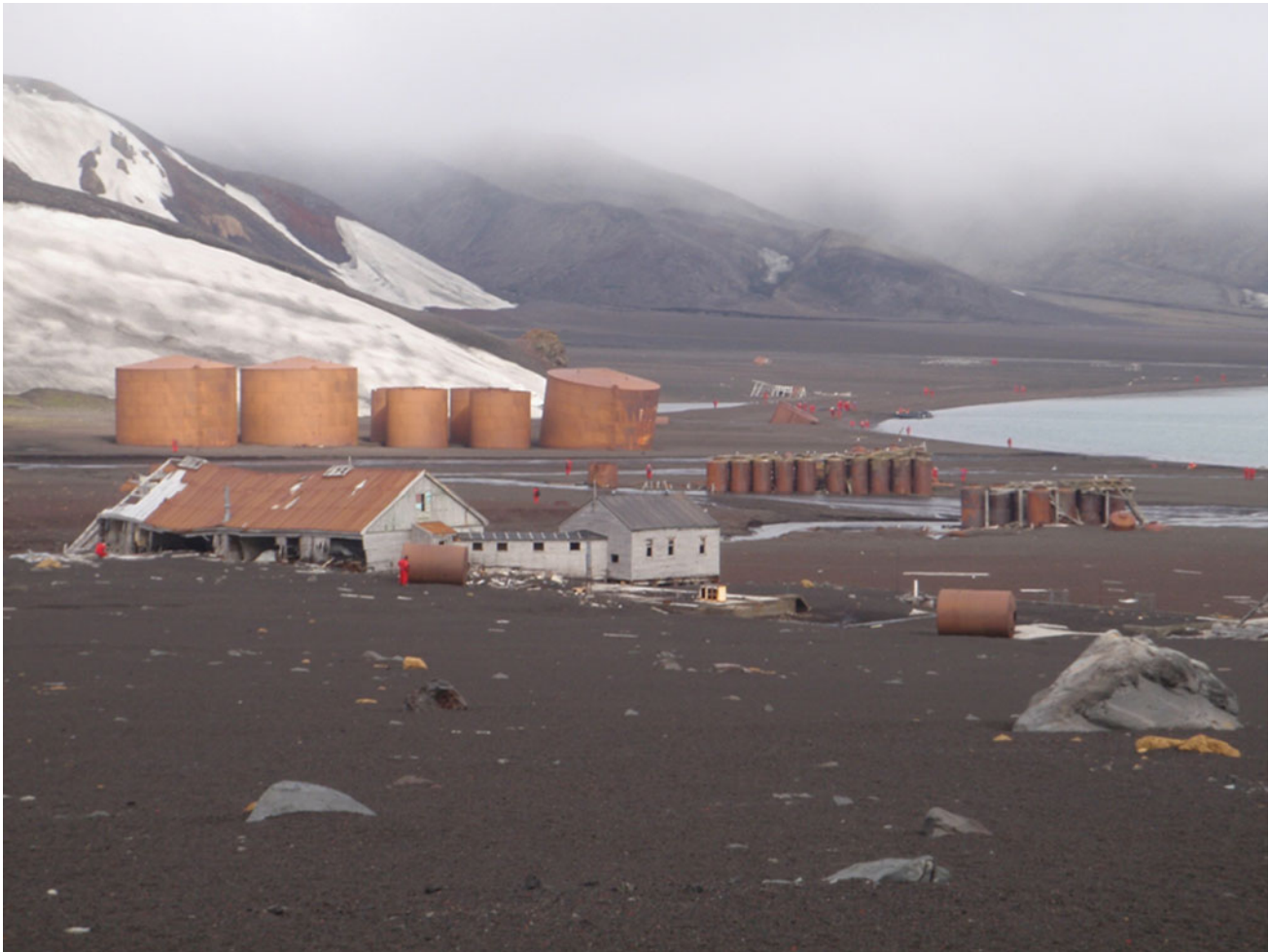
Fig. 15.2 Historic structures at Whaler's Bay on Deception Island (Photo Taken January 2013 by Tanya O'Neill)
