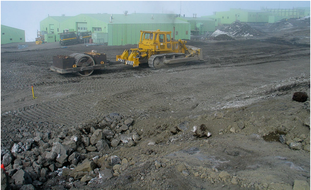
Fig. 15.3 Earth moving equipment preparing a building site adjacent to Scott Base is an example of the most intense scale of disturbance that occurs near permanent bases (Photo Taken January 2004 by Megan Balks)
