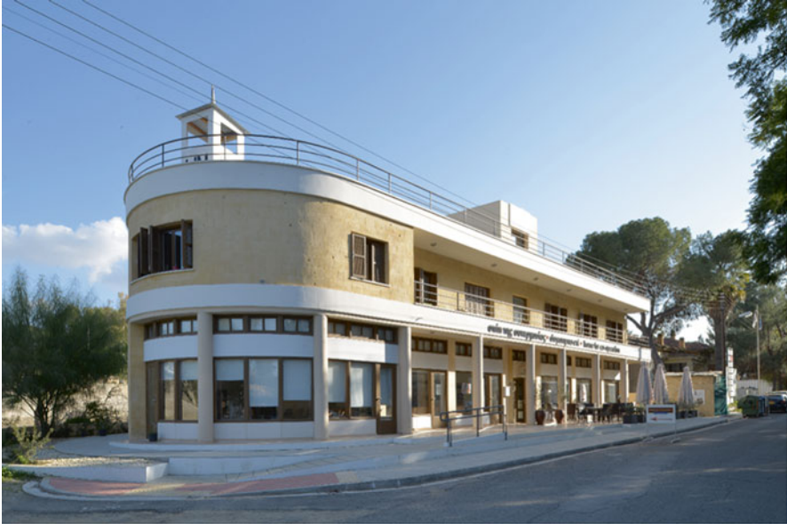
Fig. 3 The Home for Co-operation from the outside as it is today
