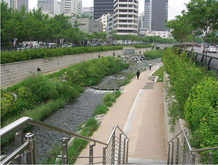
Fig. 27.2 Re-naturalised banks on the Cheonggyecheon (2003). The project aimed to construct an environment with natural habitats and clean water for the fish, birds and insects that have populated the stream excavation. The stream contributes to the reduction of temperature in the nearby areas by 3.6 °C. The decrease in traffic volumes was made possible by the implementation of public transport and the demolition of the two heavily used roads. The project has been criticised by a number of Korean environmental organisations for its high costs and from the ecological and historical point of view
