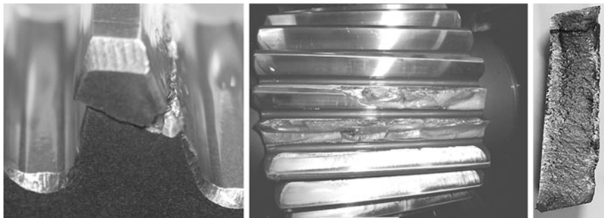
Fig. 8 Examples of flank breakage in the region of pitch diameter (Wikov MGI, a.s.)
