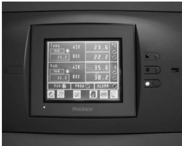
Fig. 7 Display with humidity and temperature
