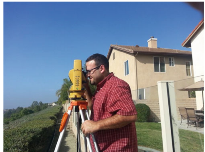
Fig. 8 Field surveying to prepare the cross-section of the slope
