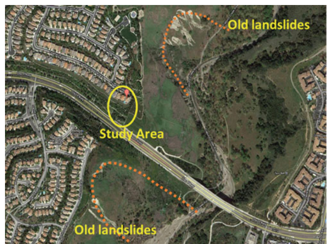
Fig. 2 Google earth image of the study area—two existing landslides are clearly visible in the area
