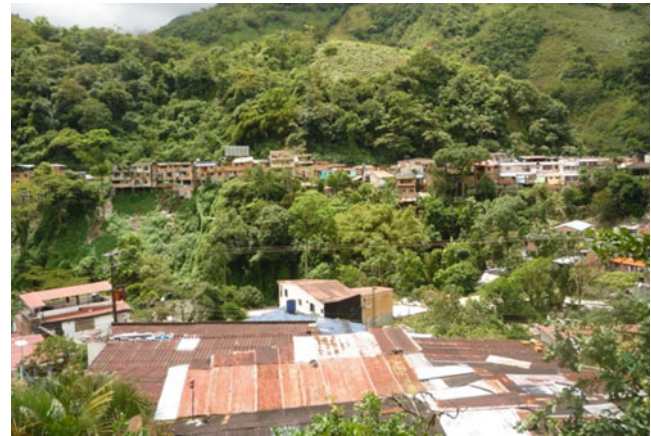
Fig. 8 Guayabetal municipality: unstable vegetated slopes
