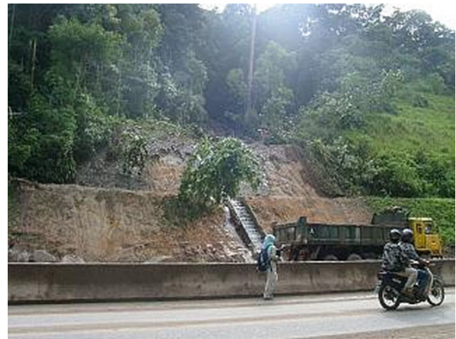
Fig. 2 General view of the debris flow at Lentang
