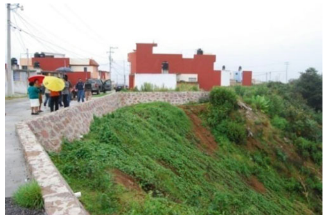
Fig. 3 Slope monitoring site, San Andrés borough
