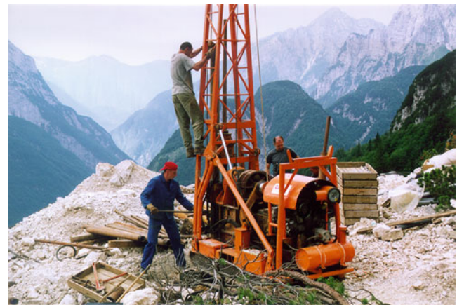
Fig. 1 Drilling work for a borehole (piezometer) above the scarp of the Stože Landslide in NW Slovenia
