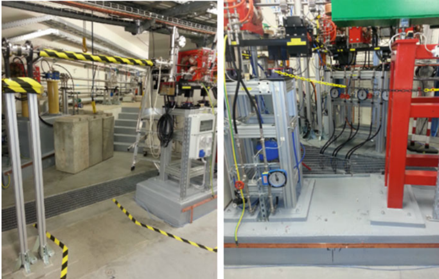
Fig. 5.4 Operating environment within industrial plant
