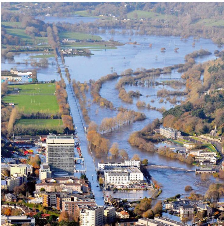
Fig. 4.18 Flood problems in Cork (Courtesy: Irish Examiner)
