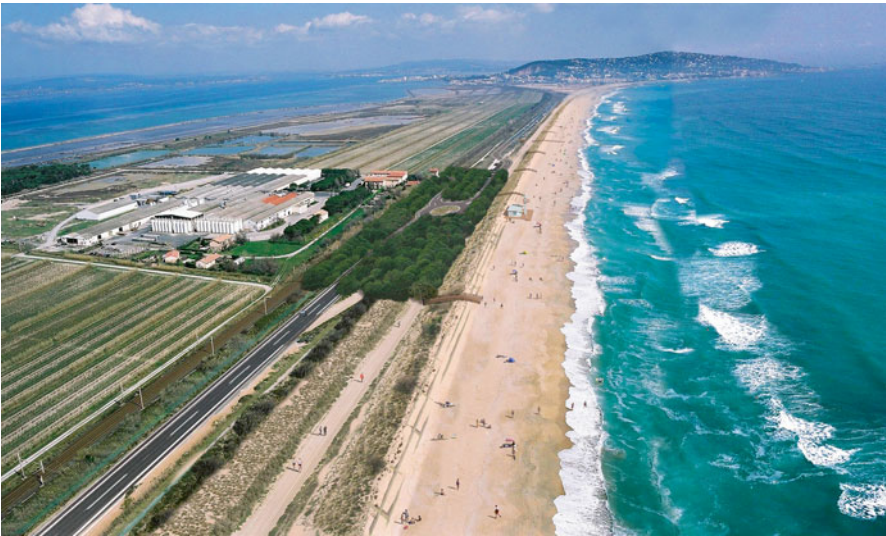
Fig. 4.21 Global overview after completion of the project showing the road moved inland and the restoration of a wider beach and sand dune
