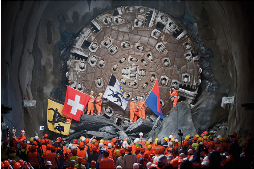
Fig. 5.2 Breakthrough in the Gotthard Tunnel 15 October 2010 ( Source Alptransit)
