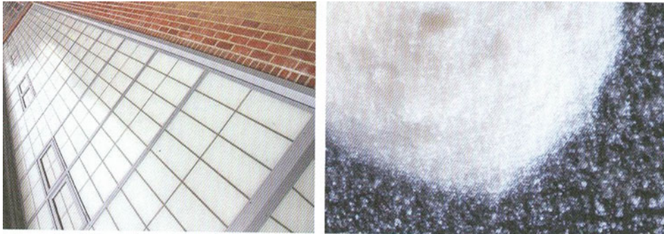
Fig. 44.2 Transparent heat insulation for industrial buildings, aerogel structure. Source: Peters, S. 2011. p.111
