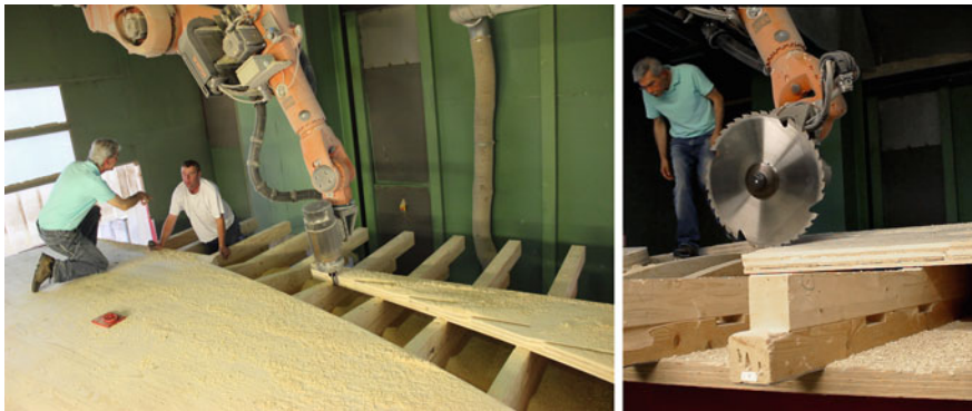
Fig. 11 Robot fabrication of the full-scale prototype. Left fabrication of the joint CV 1 -CX using a 25 mm shank-type cutter. Right formatting of the side of the panels using a saw blade with a diameter of 800 mm
