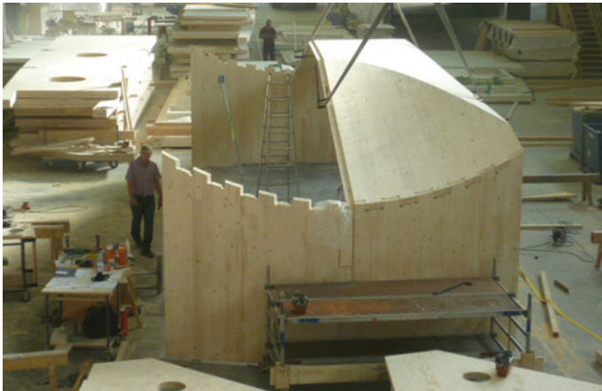
Fig. 13 Assembly of the dovetail-type connectors between the wall panels and the roof panels (Connections CV–CX)
