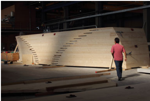
Fig. 12 Left assembly of the roof panels: shell prototype ready for the insertion of the LVL connectors (connections CV–CX). Right schematic drawing of the connector elements made from cross-laminated LVL panels. The slots have been cut with a 30 mm shank-type turn blade-knife cutter
