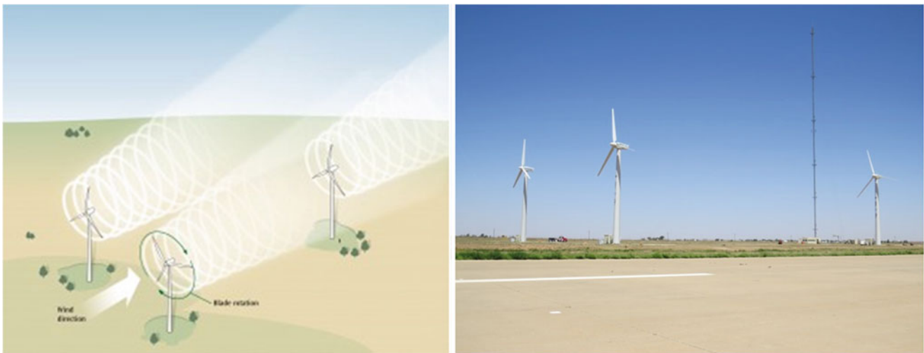
Fig. 32.1 Scaled wind farm technology facility concept ( left ) and completed construction ( right )
