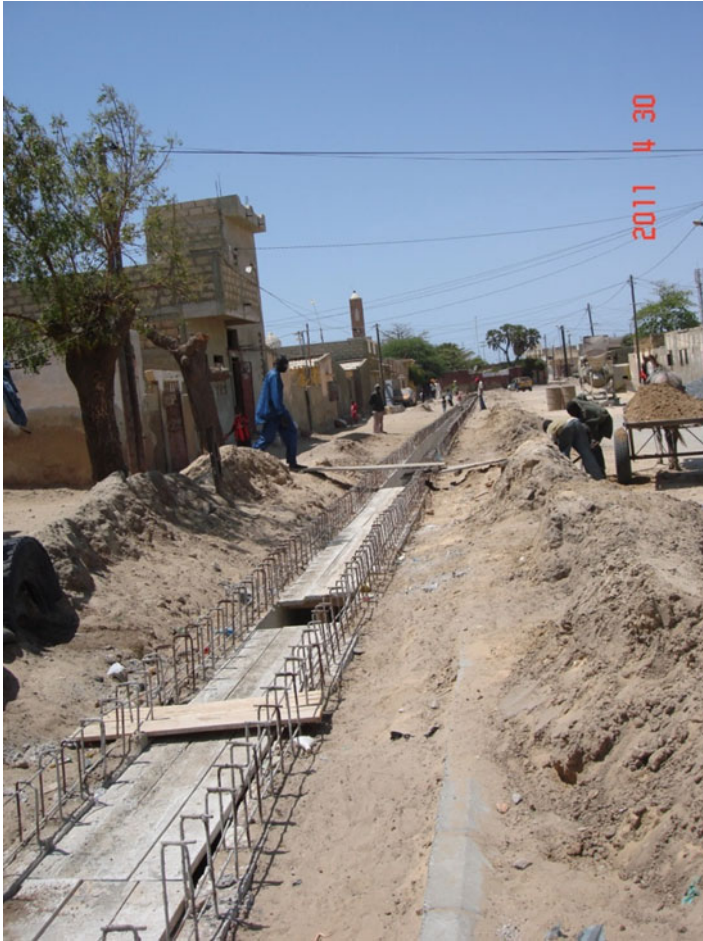
Fig. 9.5 Construction of new drains and sewerage in Diaminar (Picture: Trond Vedeld 2012)
