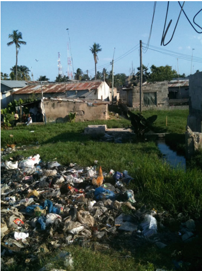
Fig. 9.3 Drains blocked by solid waste in Bonde la Mpunga (Picture: Trond Vedeld 2012)
