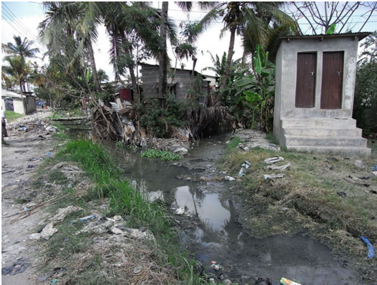
Fig. 6.7 Elevated toilets next to a clogged drain (Picture: Sigrun Kabisch 2012)
